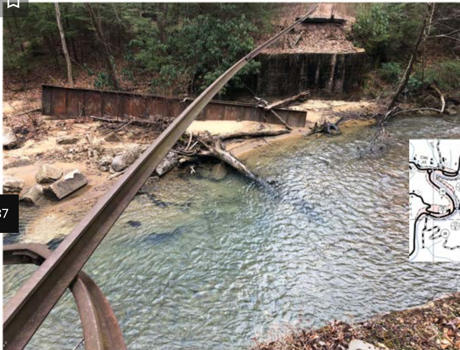
FLOOD REPAIRS ALONG THE BUFFALO CREEK & GAULEY RAIL TRAIL
