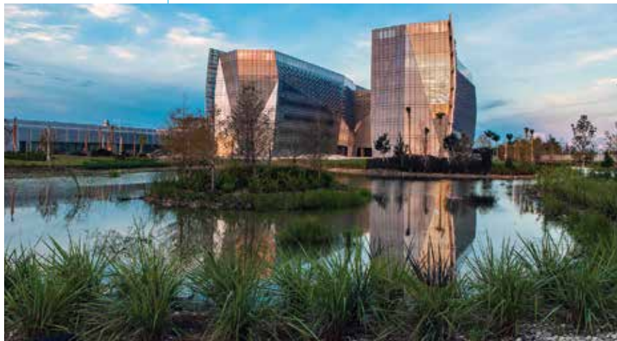
ABOVE In Florida, constructed wetlands at the Miramar FBI building are prime pollinator breeding grounds.
